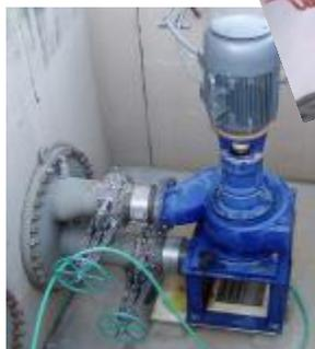
SPAD acting as flow switch, plumbing Flow Switch disconnected. Flow indicator to controller when pump is powered ON.
